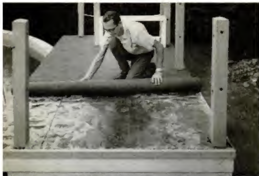
INDOOR-OUTDOOR CARPETING insures skidproof footing, goes over 15-lb. felt and 6-mil polyethylene
